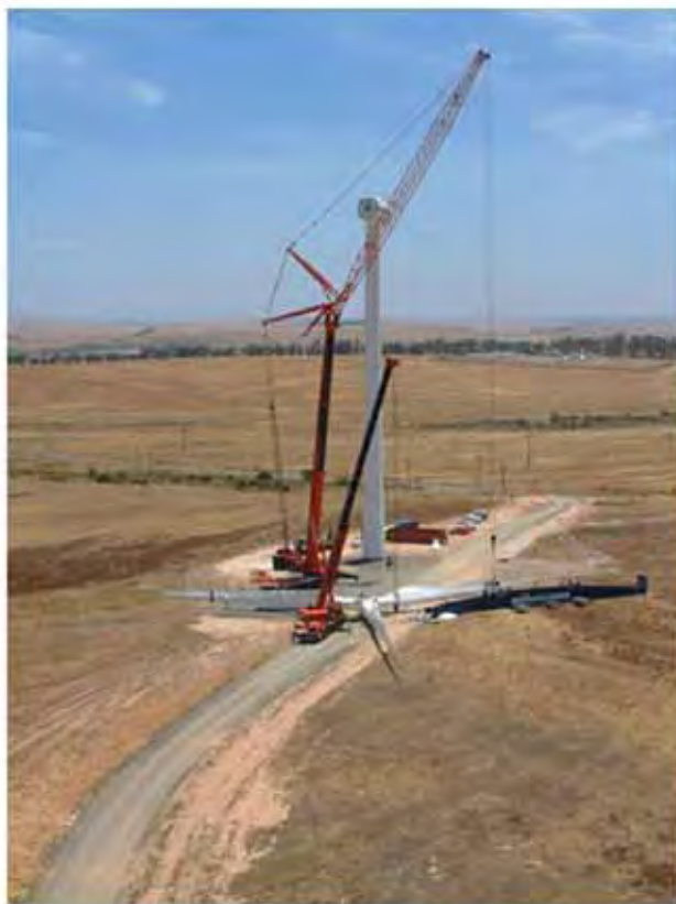
Figure 3.3: Photograph illustrating the laydown areas required during the erection of one of the turbines at the Klipheuwel demonstration facility (photo courtesy of Eskom)
