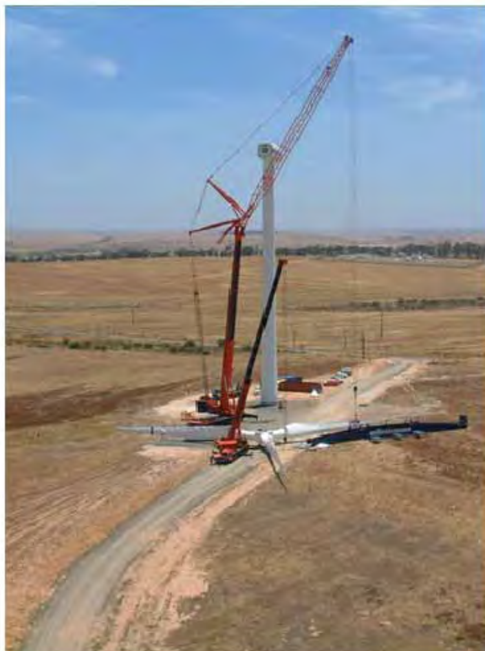
Figure 3.5: Photograph illustrating the laydown areas required during the erection of one of the turbines at the Klipheuwel demonstration facility (photo courtesy of Eskom)
