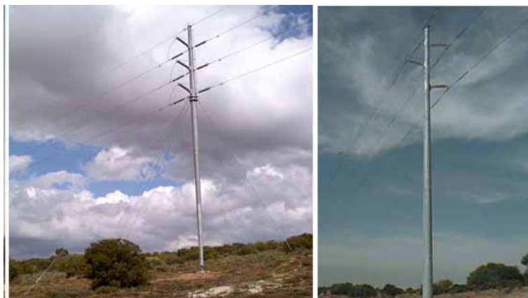
Figure 3.6: Examples of the proposed 132 kV monopole double and single circuit power line tower type
