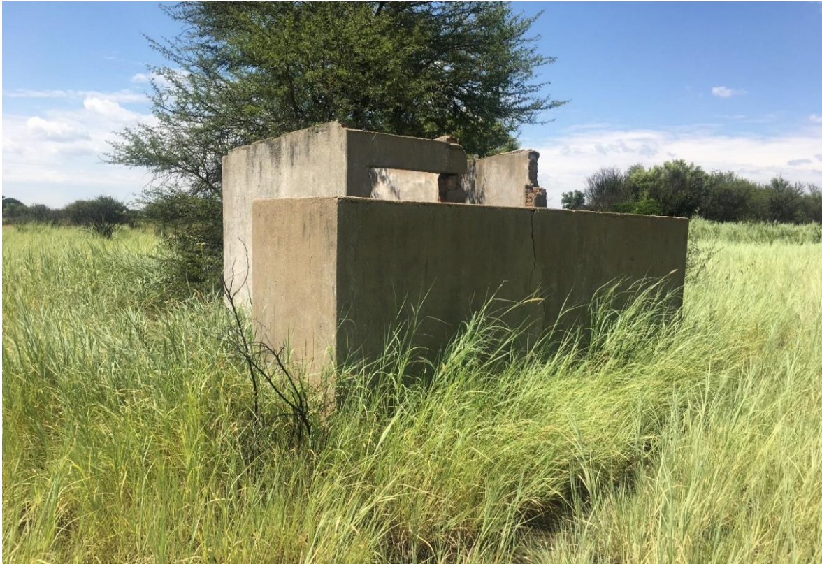
Figure 14: Structure noted on the proposed area.
