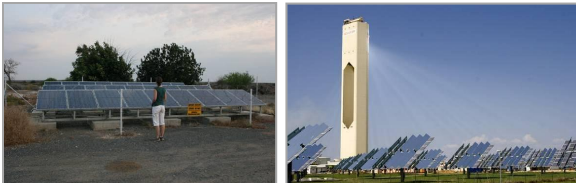
Figure 2-7: Photovoltaic solar cells (left) 23 and a CSP system (right) 24 were considered for the proposed PV plant
