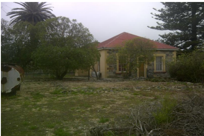
Figure 2 SOUTH ELEVATION OF HOUSE38
