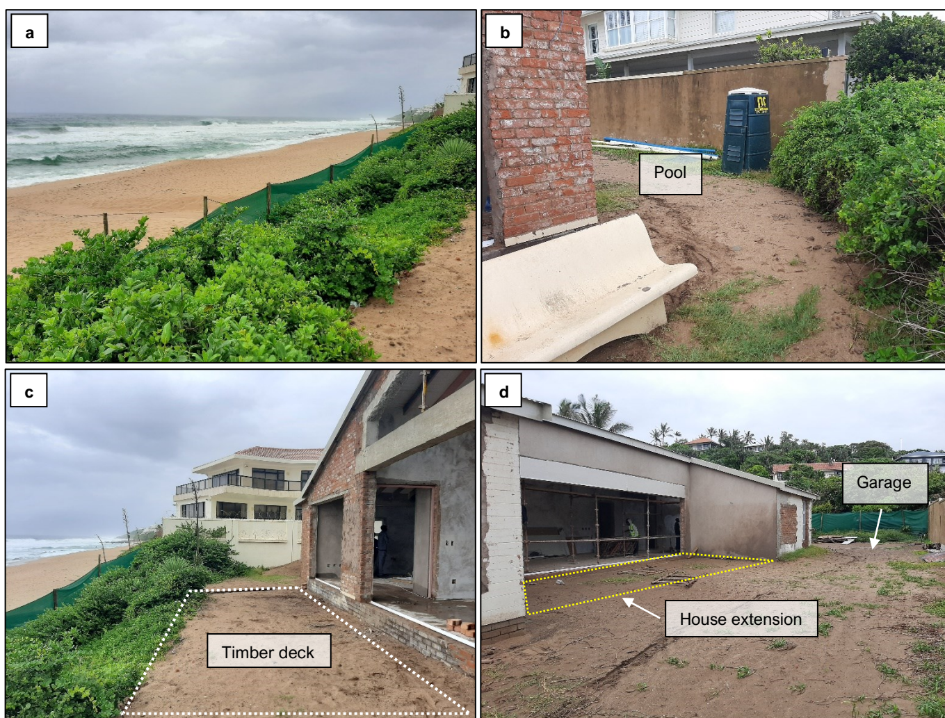
Figure 7: Photographs Showing the Characteristics of the Site Taken on the 25 th January 2021: (a) Dune in front of the existing house where the geofabric wall will be established; (b) Photograph of the northern property boundary showing the location of the proposed swimming pool; (c) Front of existing house where the timber deck will be constructed; and (d) Northern side of the house showing the proposed new house extension and new garage to be constructed towards the back of the property.
