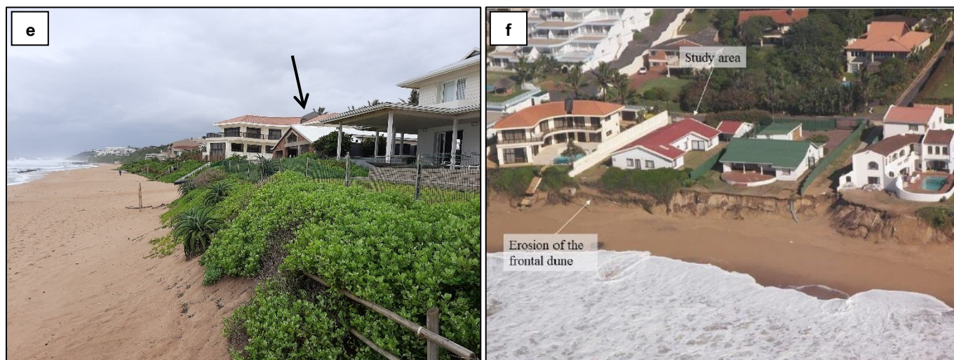
Figure 7 (cont.): Photographs Showing the Characteristics of the Site Taken on the 25 th January 2021: (e) Black arrow indicating the location of House Gotz and the surrounding beach environment; and (f) Historic image of the study area taken after the 2007 storm event showing erosion of the dune (source: SDP, 2021).
