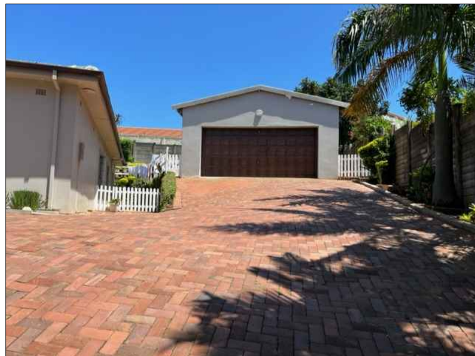
View of Existing Garage & Driveway
