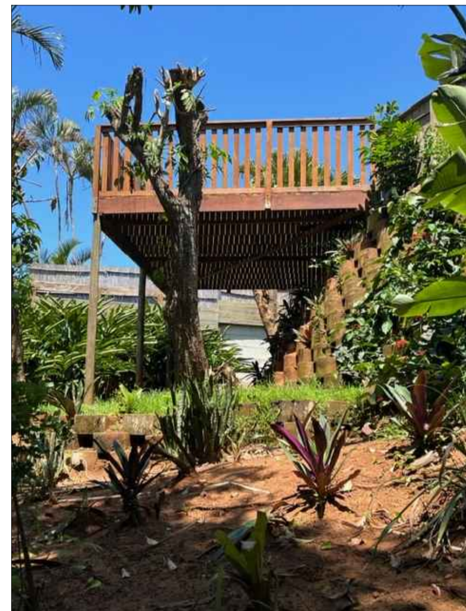
View of new Timber Deck & Retaining Wall
