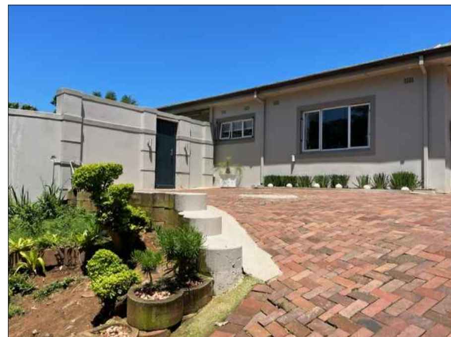
View of new wall and gate to Pool Area
