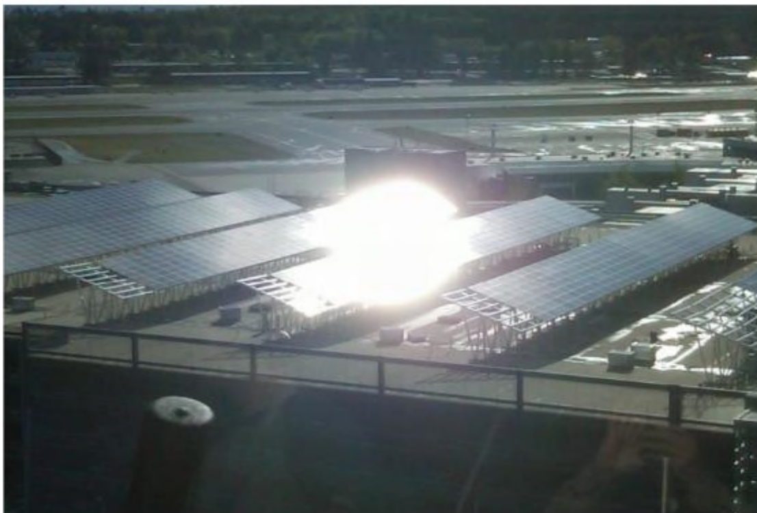
Plate 7 - Glare experienced in the Control Tower at Boston Regional Airport from a PV array
