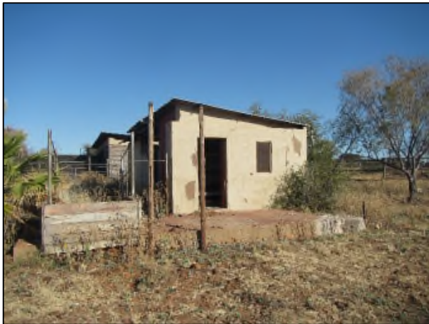
Figure 40: The earliest house on the property at waypoint 1161.
