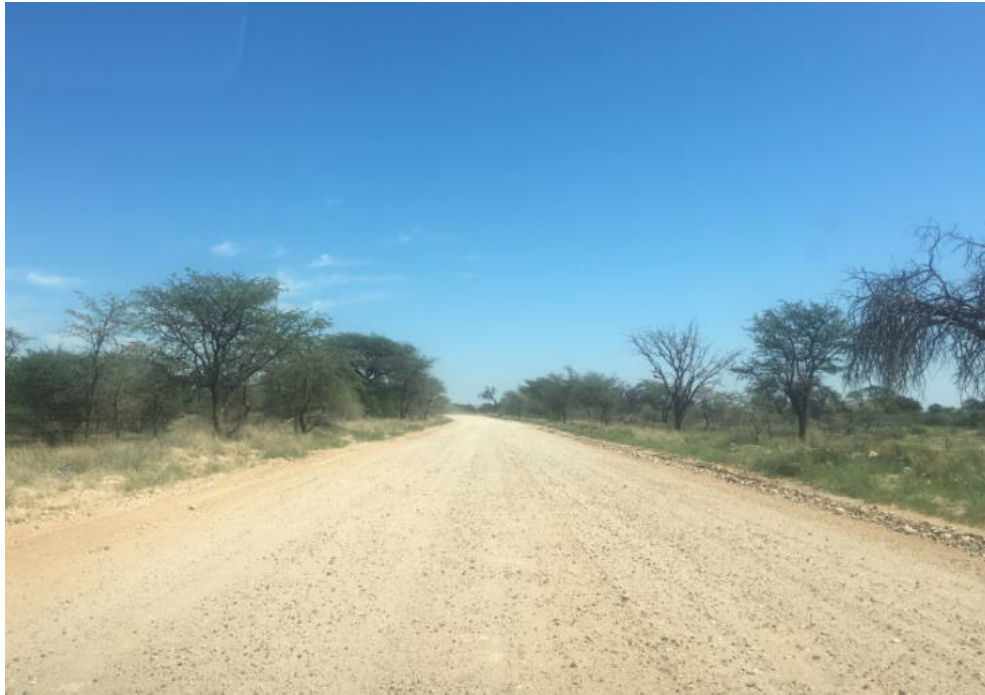
Figure 11: Existing T25 gravel road
