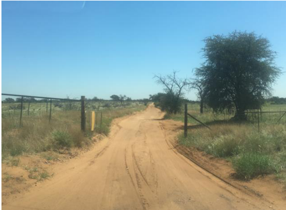
Figure 8: Existing T26 gravel road
