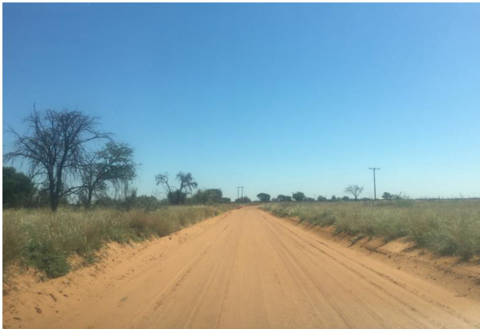
Figure 9: Existing T26 gravel road
