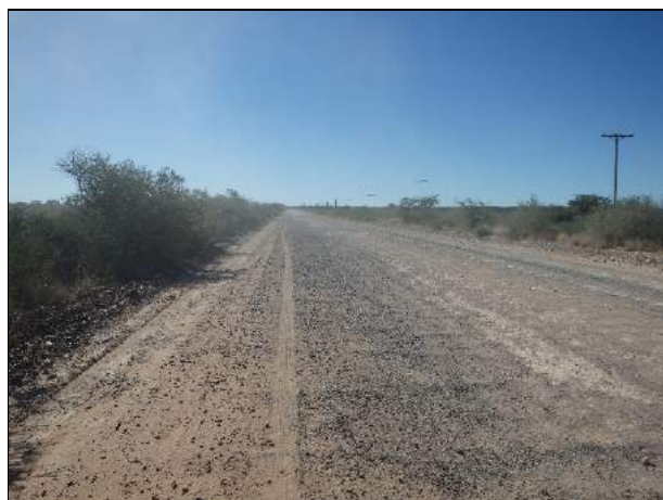
Figure 1: Photograph of the existing T25 gravel road. Several pan wetlands were identified within its 500m investigation area, the closest being approximately 45m from this road (Pan Wetland 8).
