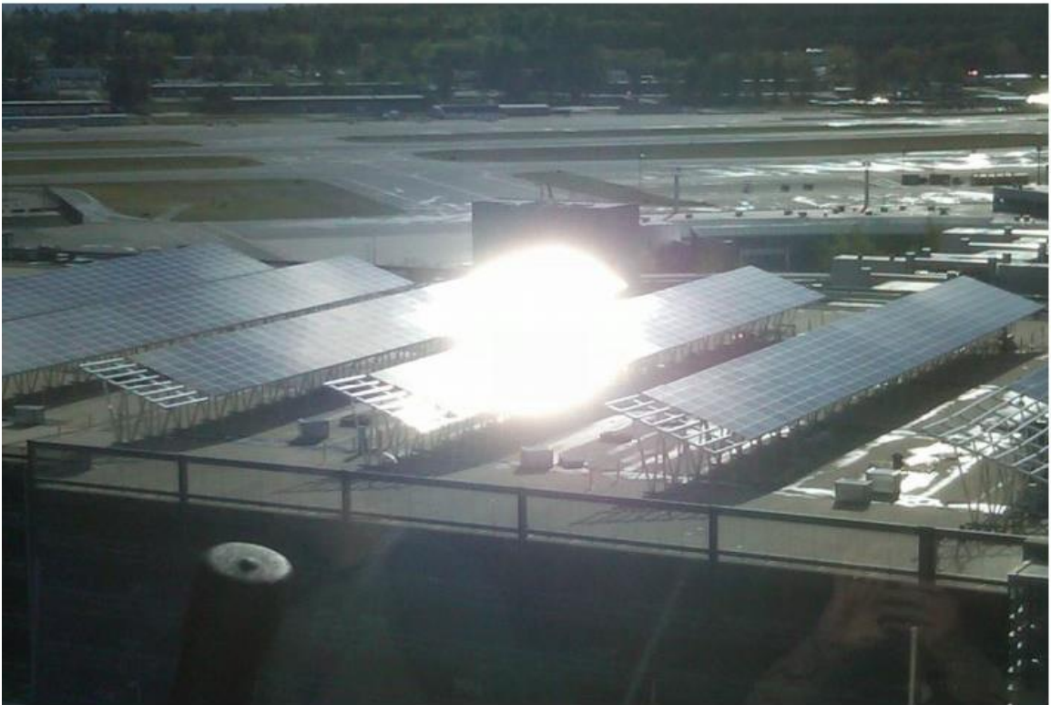
Plate 3, Glare experienced in the Control Tower at Boston Regional Airport from a PV array
