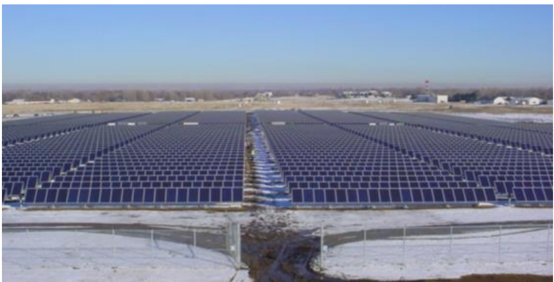
Plate 2, PV array viewed from above. Note the array rows are read as one and have a similar impact as the roof of a large industrial building might.
