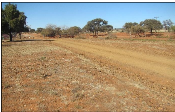
Figure 14: View along access road Alternative 1 towards the southeast.
