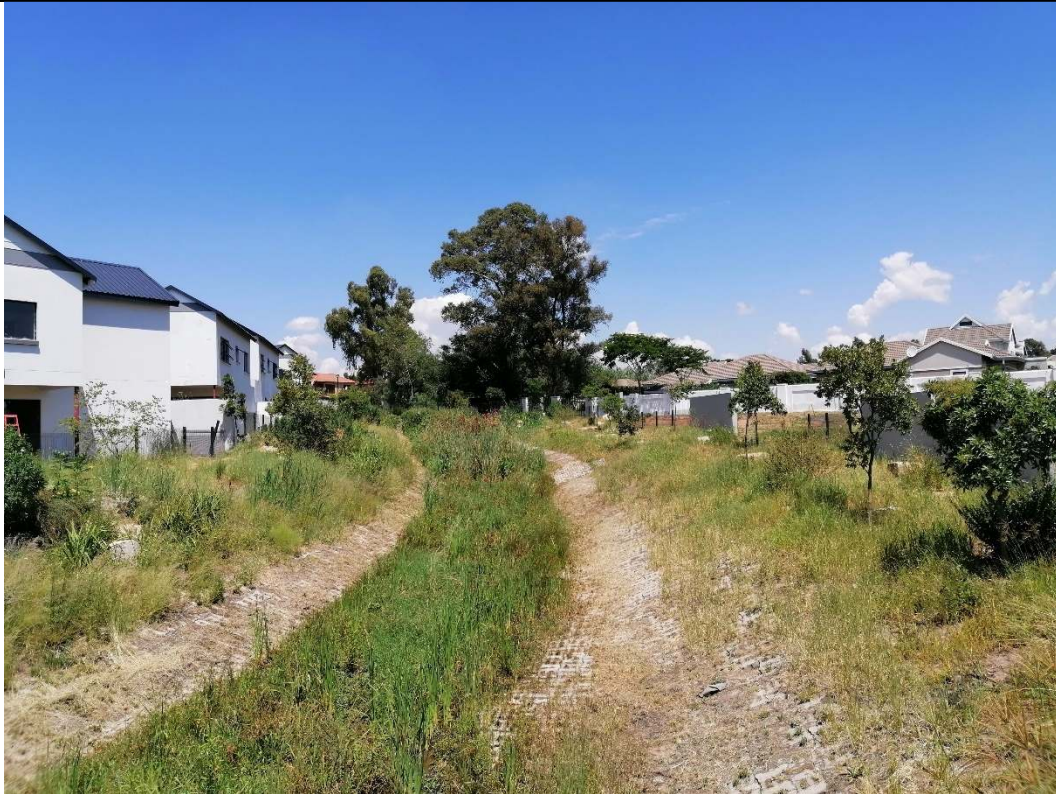
Adjacent development to the west including bio-engineered stormwater channel (seen from in Kengies Extension 40)
