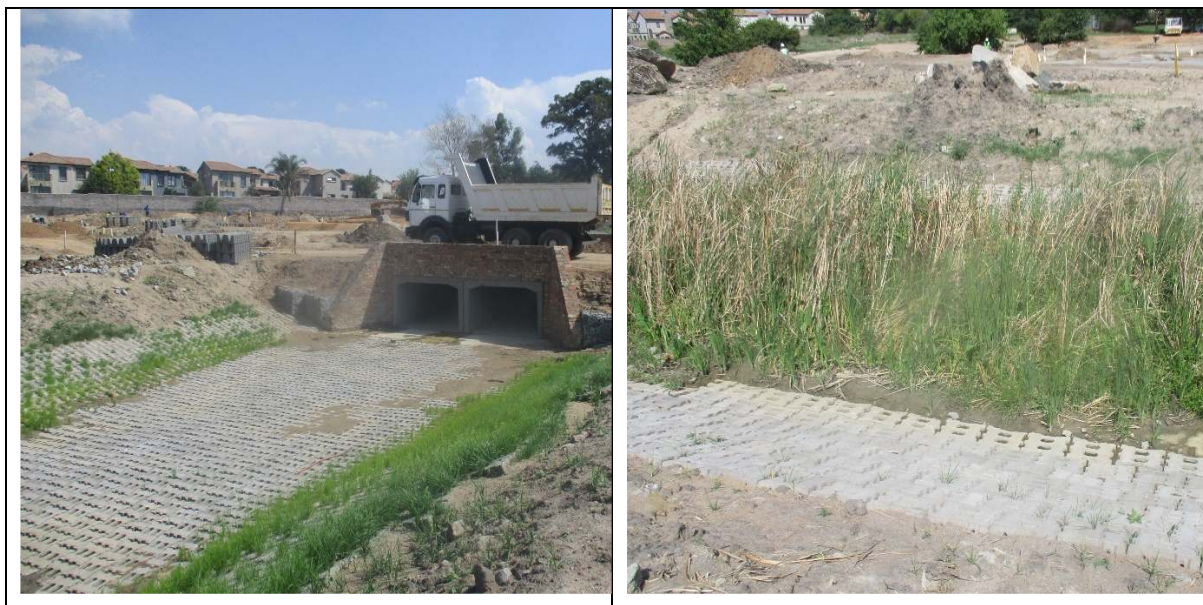
Figure 4-11: Photograph of armoflex channel on adjacent property
