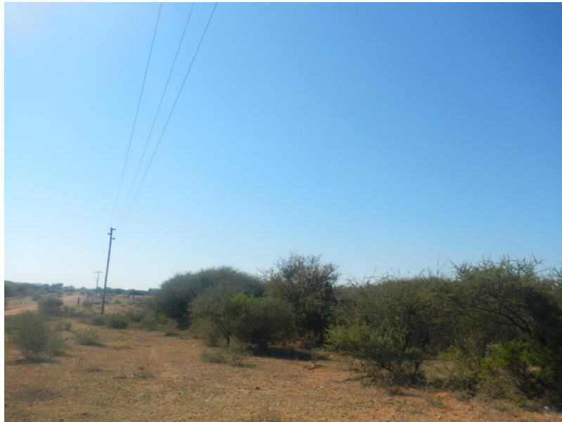
Figure 19: Power line traversing across the proposed development site
