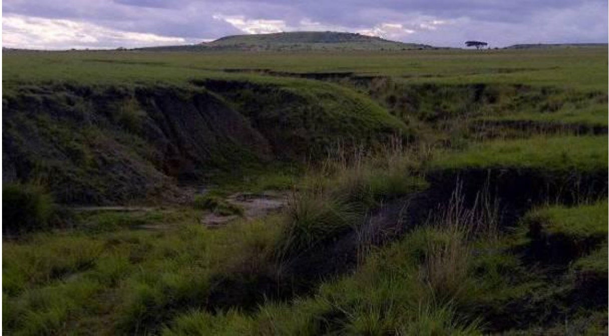
Fig 5 Eroding river banks and riparian area
