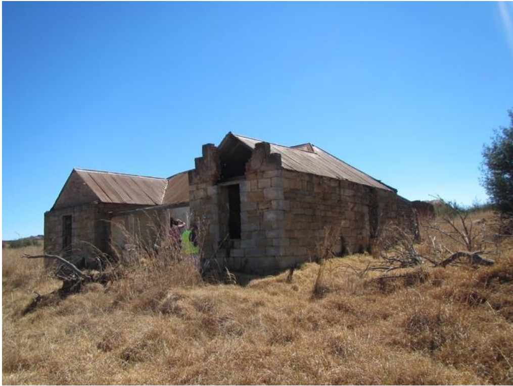
Historic sandstone structure
