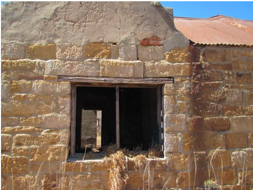
Historic sandstone brick structure
