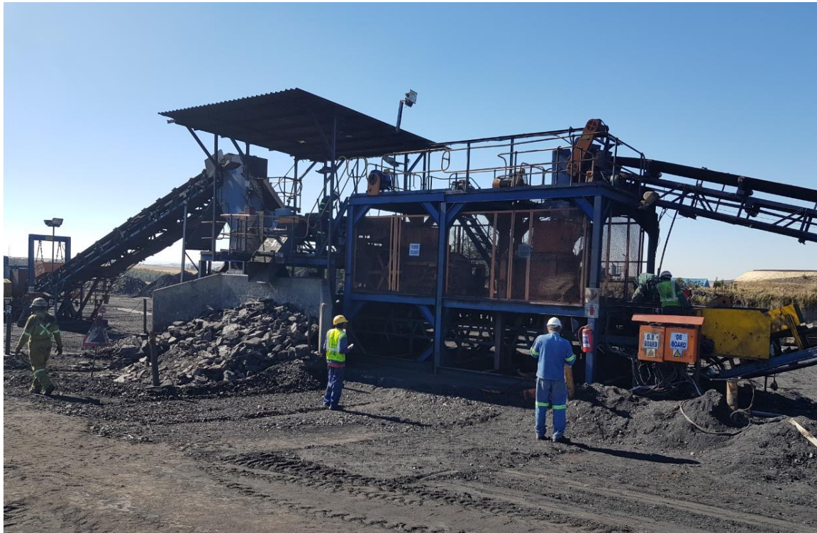
FIGURE 3-3: EXAMPLE OF A TYPICAL WASH PLANT
