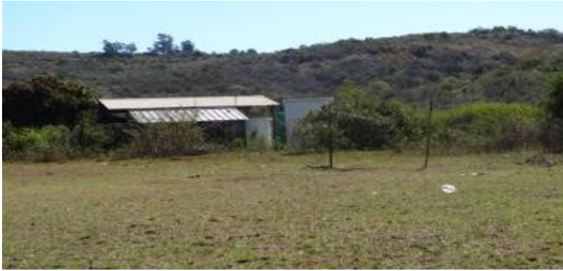
Existing water treatment facility from where the pipeline will begin.
