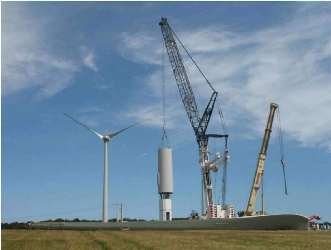
Figure 2-9: Assembly and erection of the tower sections
