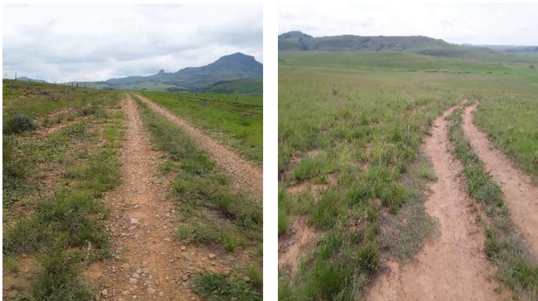
Figure 6: Vie of some of the access roads within the site
