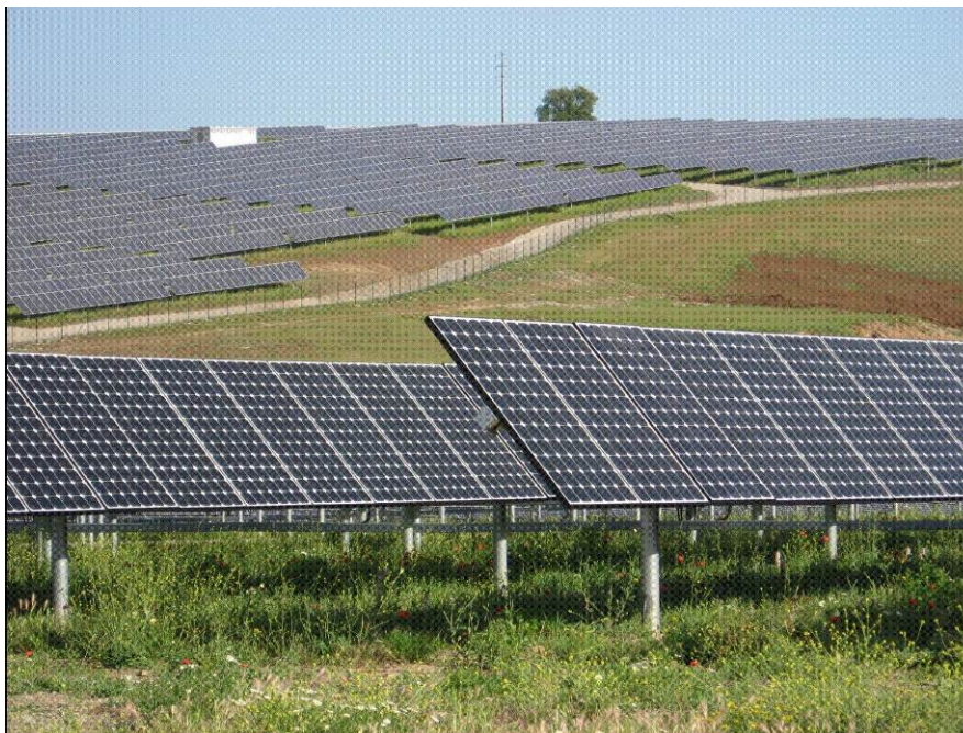
Figure 3: Illustration of a photovoltaic solar energy facility
