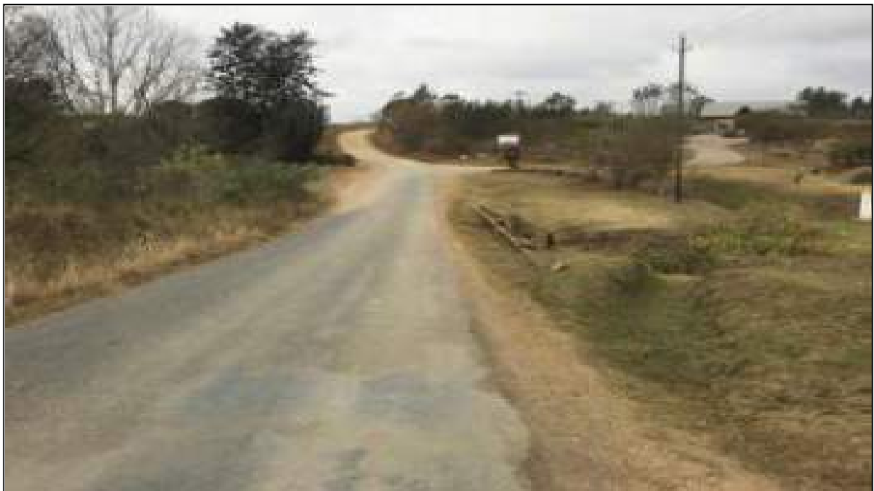
Plate 2: The Intaba Ridge access road through the Bisley Valley Nature Reserve.
