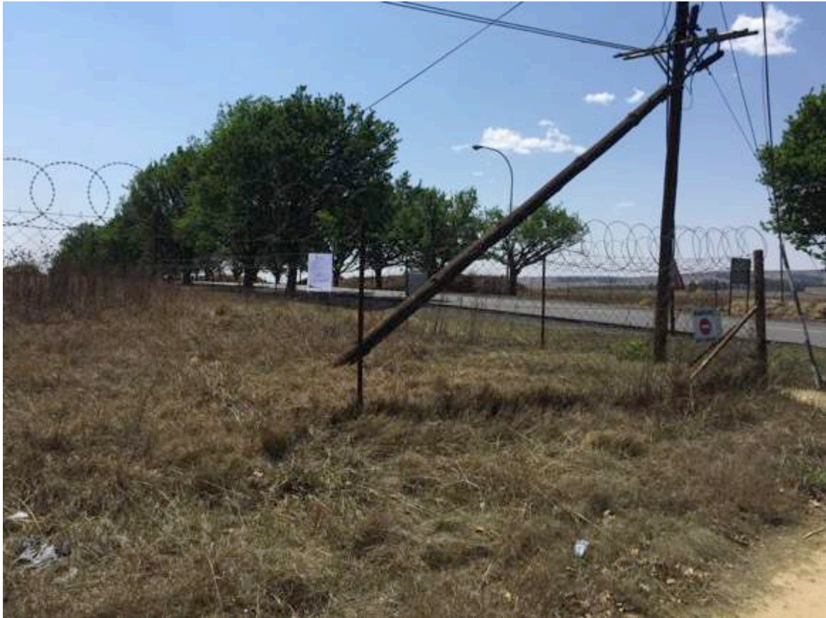
Figure 48. Sign at entrance to Camden Power Station
