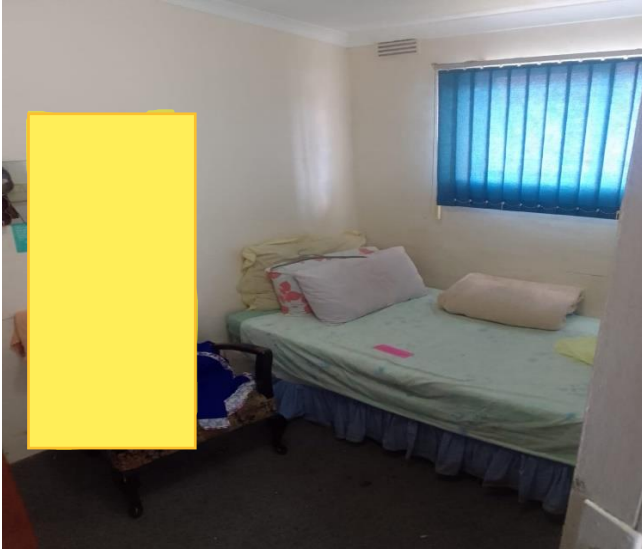
Image 1: Existing Domestic room to be converted into storeroom. Existing door to be bricked up & a new opening to be created where the yellow highlighted block is shown.
