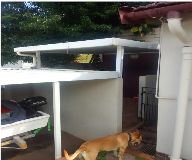
Image 3: External pic of the refuse area to be converted to domestic room
