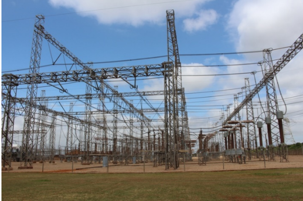
Plate 1 Sub-station busbars
