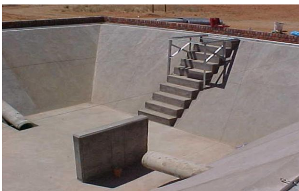
Plate 5 Oil holding dam
