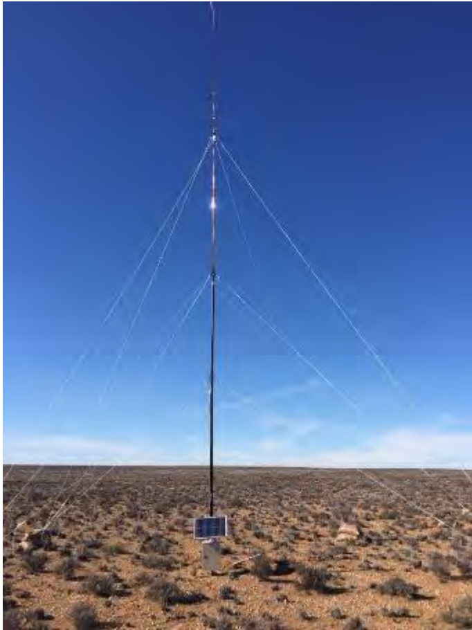
Figure 3: Short mast monitoring system
