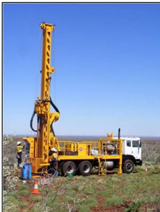
Figure 3-1: Example of a typical diamond drill rig
