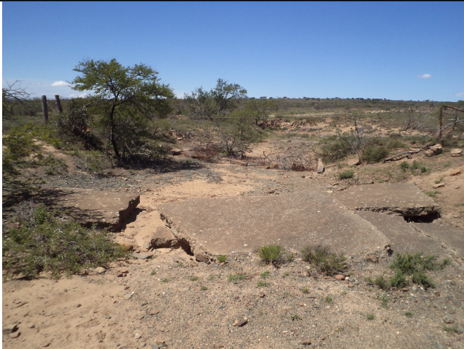
Figure 1.1: Watercourse crossing point 1 (WC1).
