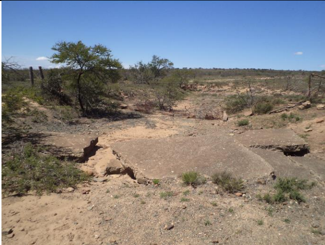
Figure 1.1: Watercourse crossing point 1 (WC1).
