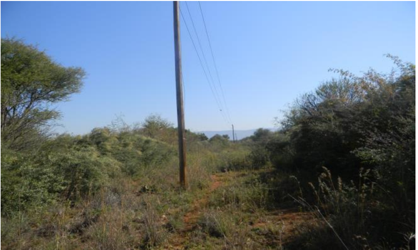
Plate 26: Photo 26: View of 22kv powerline route that cuts across the overburden site (Photograph © by Author 2016)
