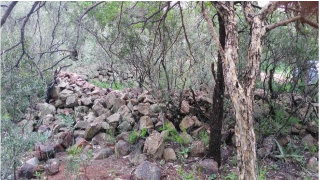
Plate 6: Photo 6: View of partial destroyed LIA stone walled stone structure near starting point of the proposed haul road (Photograph © by Author 2016).
