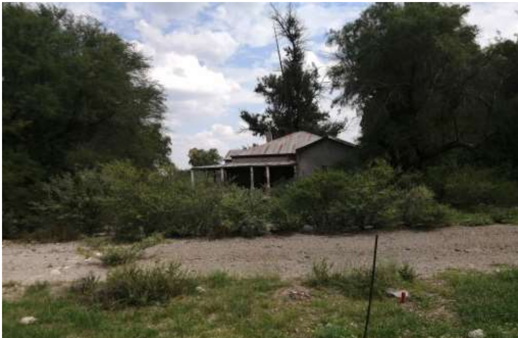
Figure 13: Old farm house on farm Uikijk 231
