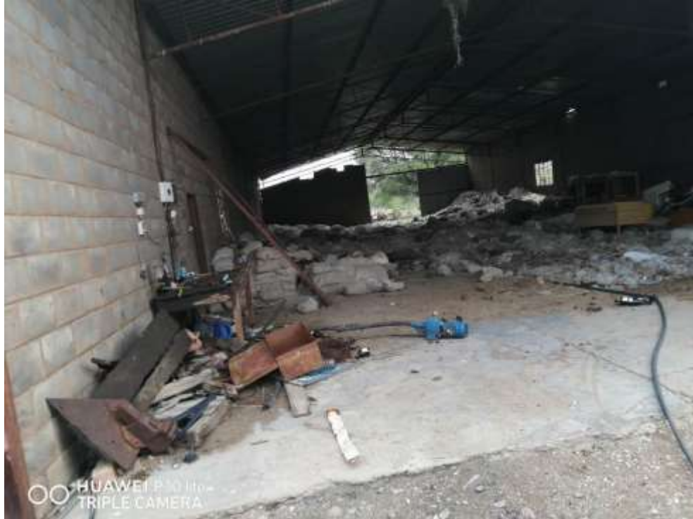
Figure 13: Waste separation plant on farm Uitijk 231
