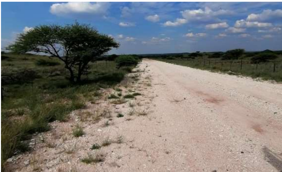
Figure 15: Existing main gravel road
