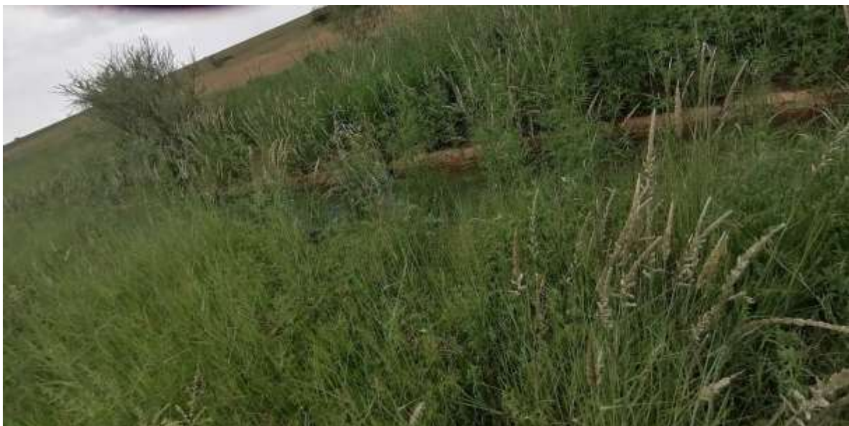
Figure 2: Cemented canal traversing over farm Kalkfontein 11
