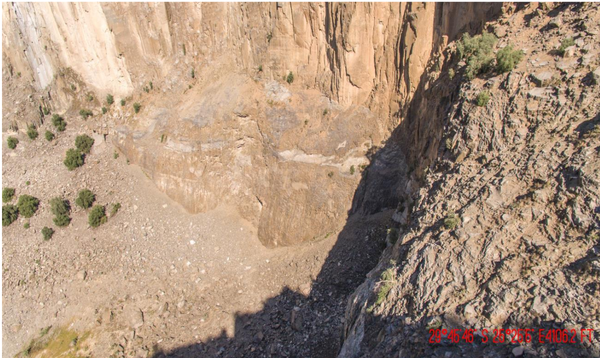
Clear indication of Pit caving in
