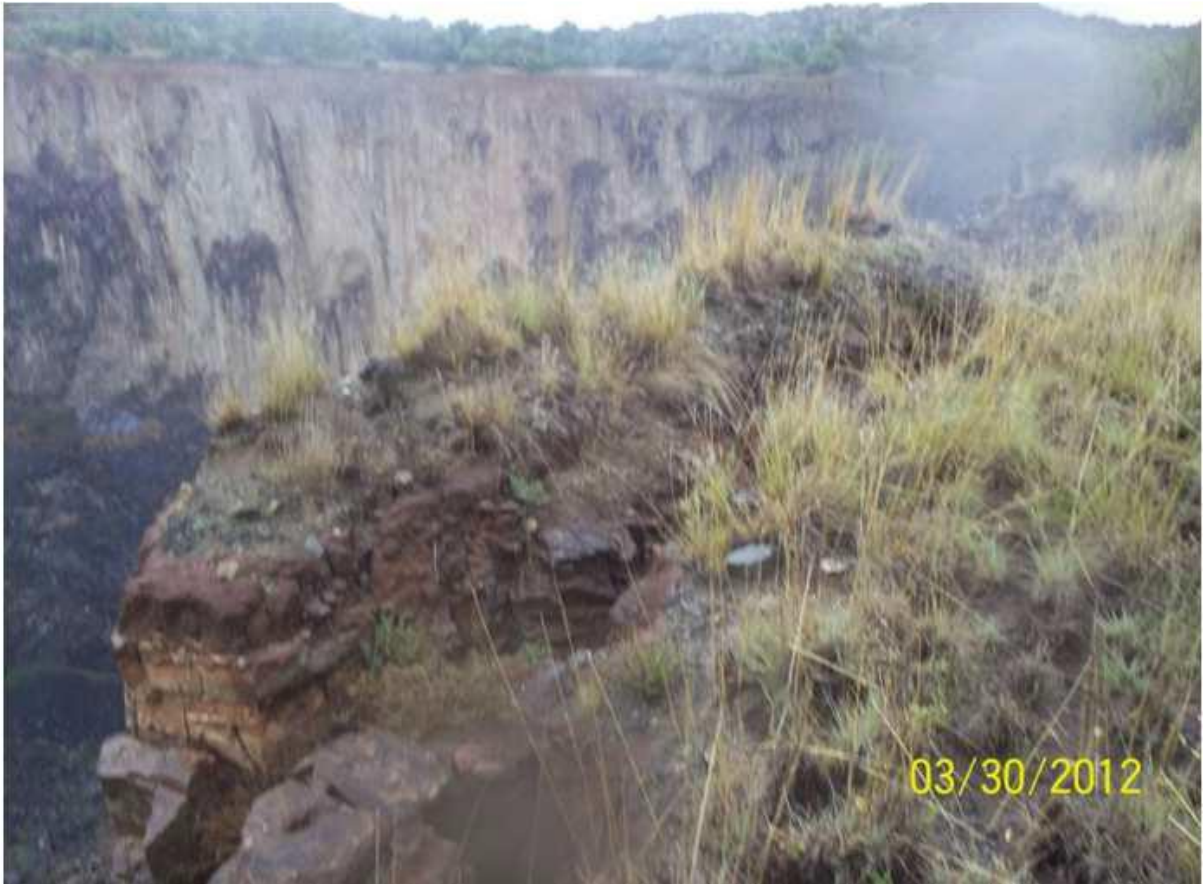
Figure 6: Block of material about to fall into the Pit.
