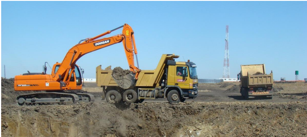
Figure 4.8.2.3 (a): Excavator and Transport Tipper Trucks
