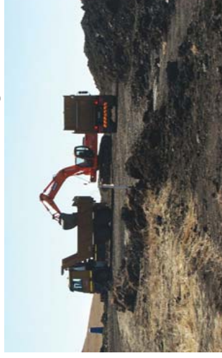
Figure 2: Soil stockpiles in the background, the excavated dolerite horizon in the middle and overburden in the foreground
