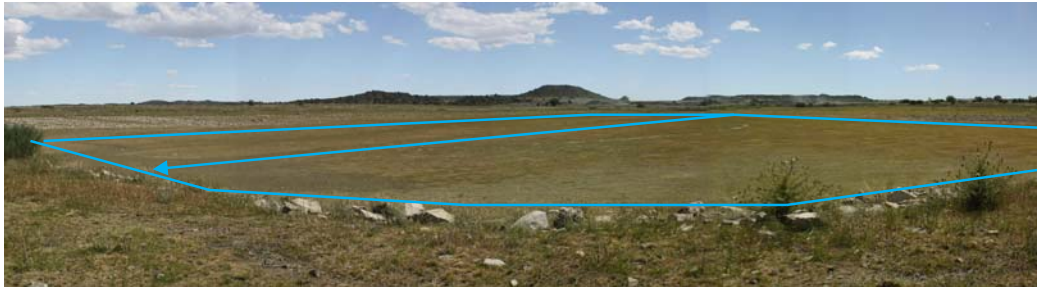
Figure 12: Panorama of the inflow of Dam 10. This area is periodically flooded and consists of an extensive wetland (blue figure). This wetland is a result of the dam and would, under natural conditions, be much smaller. The blue arrow indicates the main channel and inflow of the dam.
