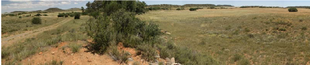
Figure 7: Panorama of the wall of a very old dam on the site. As can be seen the capacity of the dam has severely decreased due to sedimentation over the years.
