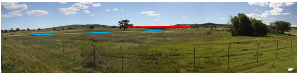
Figure 27: Panorama of the seasonal stream as it exits the mining area on the eastern border (blue line). The border of the mining area is visible as the fence line. The damwall of Dam 10 is indicated in red. This dam acts as a sediment trap and most of the suspended sediment is deposited in this dam. However, mine dumps outside the catchment of this dam releases sediment into the stream downstream of the dam.
