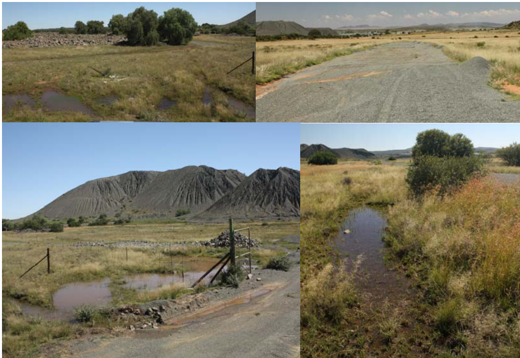
Figure 6: Selection of photographs illustrating areas where the internal road network causes ponding and erosion. This is due to the lack of culverts and the elevation of the roadways above the virgin soil level.
