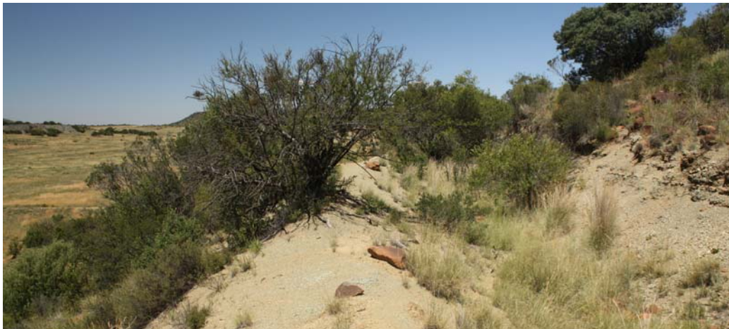
Figure 8: The surface runoff drain along the slopes of the large southern hill formation in the mining area. The drain was most probably constructed during the late 19 th century.
