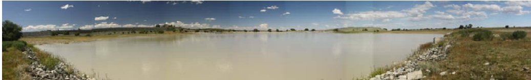
Figure 11: Panorama of Dam 10 near the eastern border of the mining area. The dam is quite large but has lost much of its capacity due to sedimentation from mine dump runoff.
