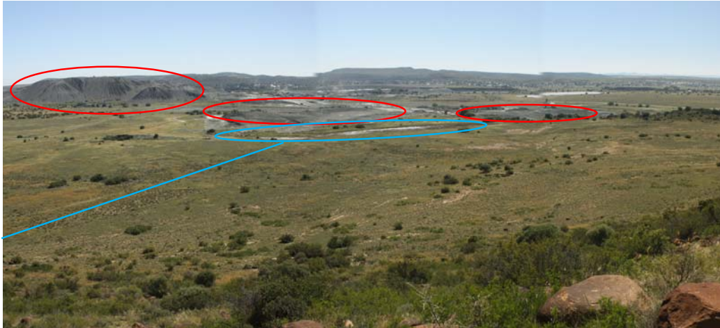
Figure 1: Panorama of mining activities on the site. Visible mine dumps are indicated (red circles). A drainage line flowing from south west has been obstructed by a mine dump and has consequently formed an artificial and degraded wetland. The drainage line and wetland is indicated in blue.
