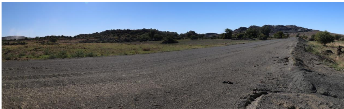
Figure 5: A few large haul roads also cause disturbance and act as flow barriers for surface runoff.
