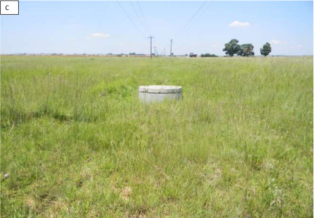
Plate 3: Photo C . showing bulkwater sewer pipeline and powerlines in the background.
