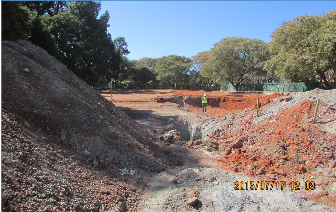
Figure 2 General view of the construction site showing one of the excavation areas in the back with two spoil heaps in the front. This photograph was taken during the site visit of 17 July 2015.
