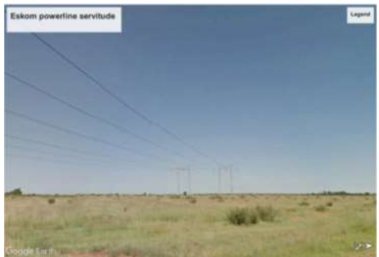
Photo 2: View of Eskom powerlines traversing the development area
