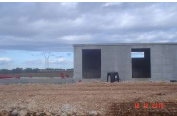
Figure 30: Typical example of auxiliary buildings under construction (Solek, 2013).
