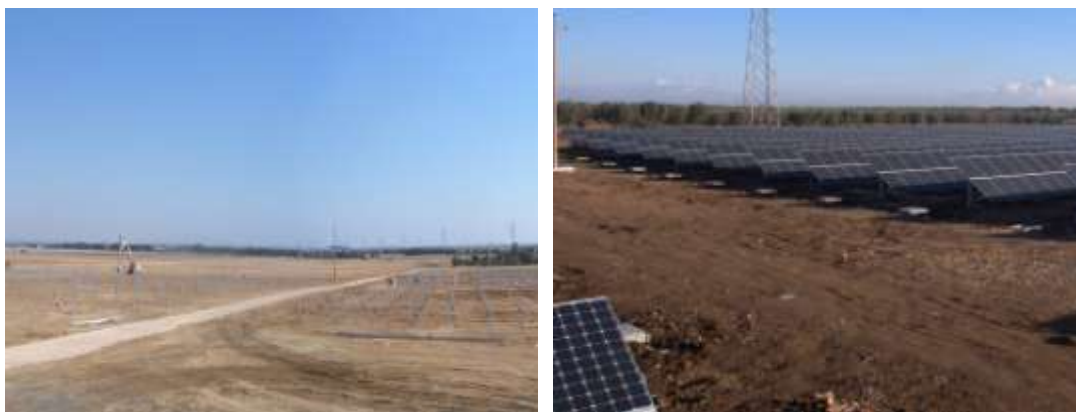
Figure 27: Showing example of typical internal roads between PV Panel Arrays (Solek, 2013)
