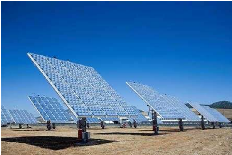
Figure 21: Example of concentrated photovoltaic (CPV) facility (Solek,2013)
