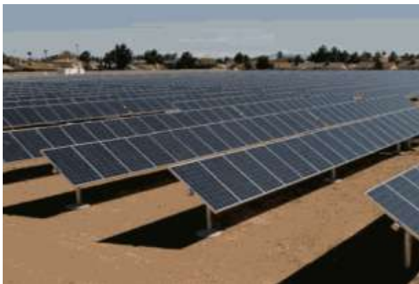
Figure 24: An example of a single axis tracking system. NB – The final tracking technology will be only be decided at a later stage during the detailed design.
