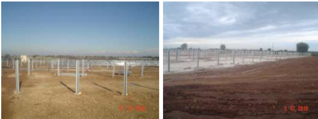
Figure 26: Showing typical examples of foundation footprints.
