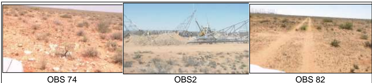
Figure 19: Photos along the route of the proposed connecting line (Lubbe,2016)
