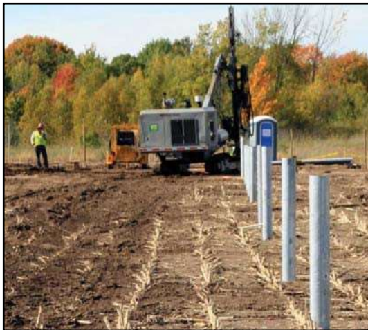
Figure 4: Driven/ Rammed Steel Pile
