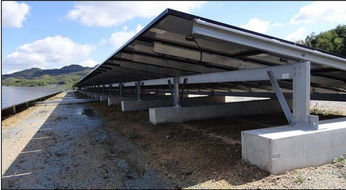
Figure 3: Cast Concrete Foundation
