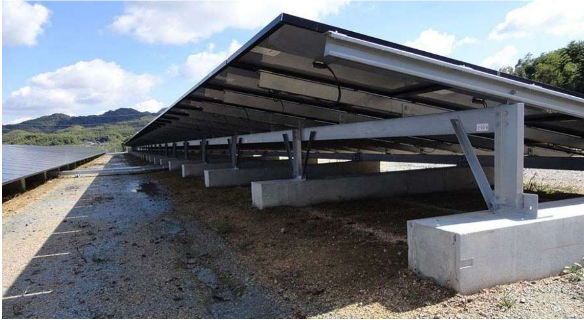
Figure 3: Cast Concrete Foundation
