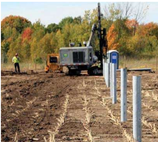
Figure 4: Driven/ Rammed Steel Pile
