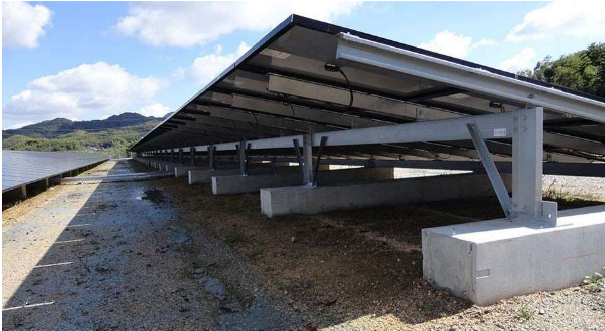
Figure 3: Cast Concrete Foundation (alternative mounting)
