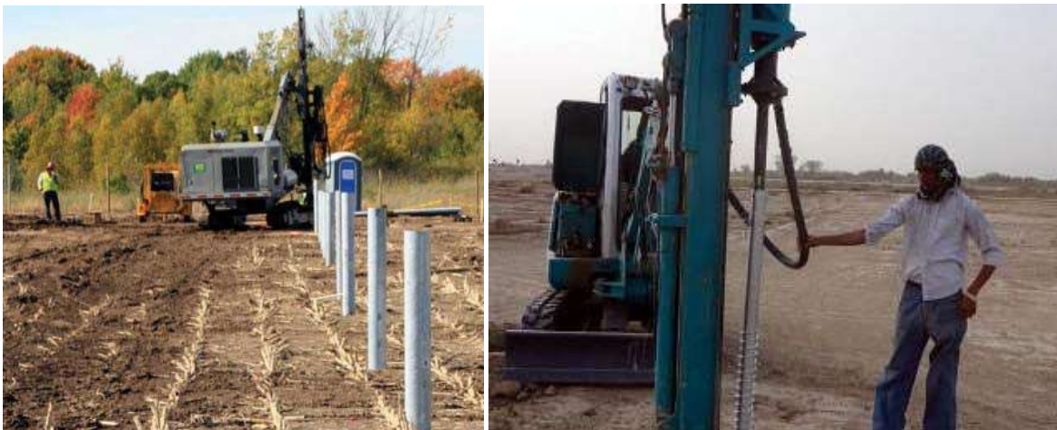
Figure 4: Driven/ Rammed Steel Pile (left) and Ground Screw (right) are the preferred mounting technology.
