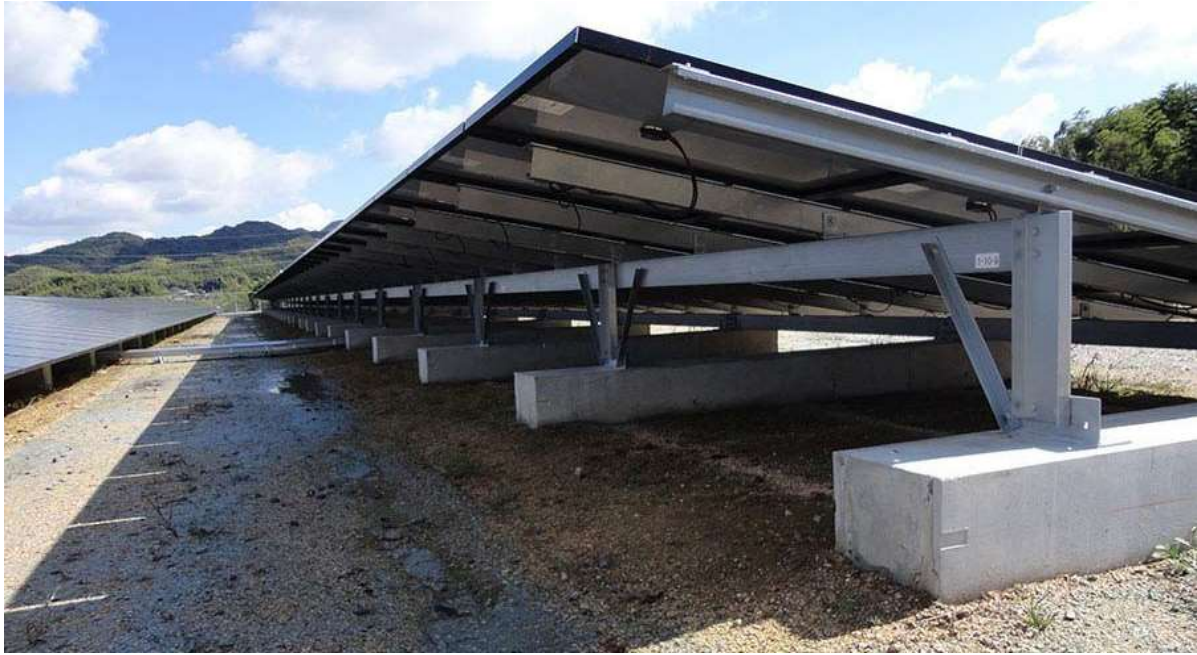
Figure 3: Cast Concrete Foundation (alternative mounting)
